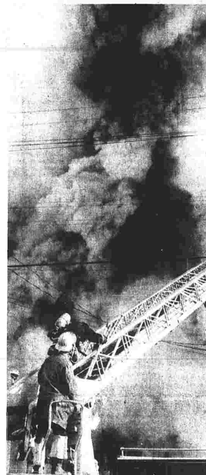
An early morning fire that gutted a store-apartment three-story building on Union Street in Rockville. The fire produced billows of thick black smoke and left five families homeless. Several firefighters and two children who lived in the building were brought to the Rockville General Hospital for emergency treatment of minor injuries and smoke inhalation. (Herald photo by Richmond)
